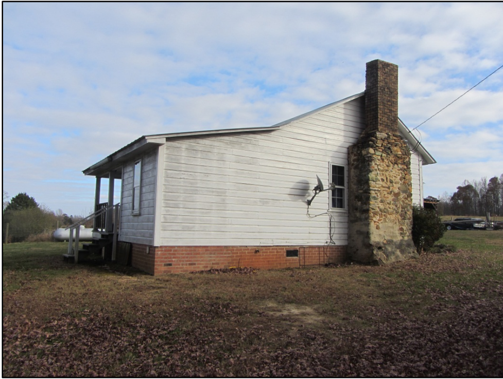
Figure 25. Ward Mill House (AM 458), west elevation, looking east from mobile home.
