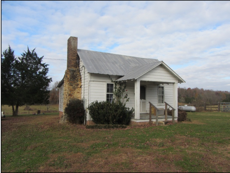
Figure 24. Ward Mill House (AM 458), south façade, looking north from driveway.
