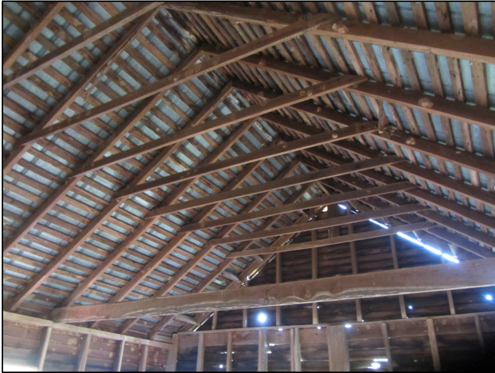
Figure 19. Ward Mill (AM 457), interior view of roof system, looking south.
