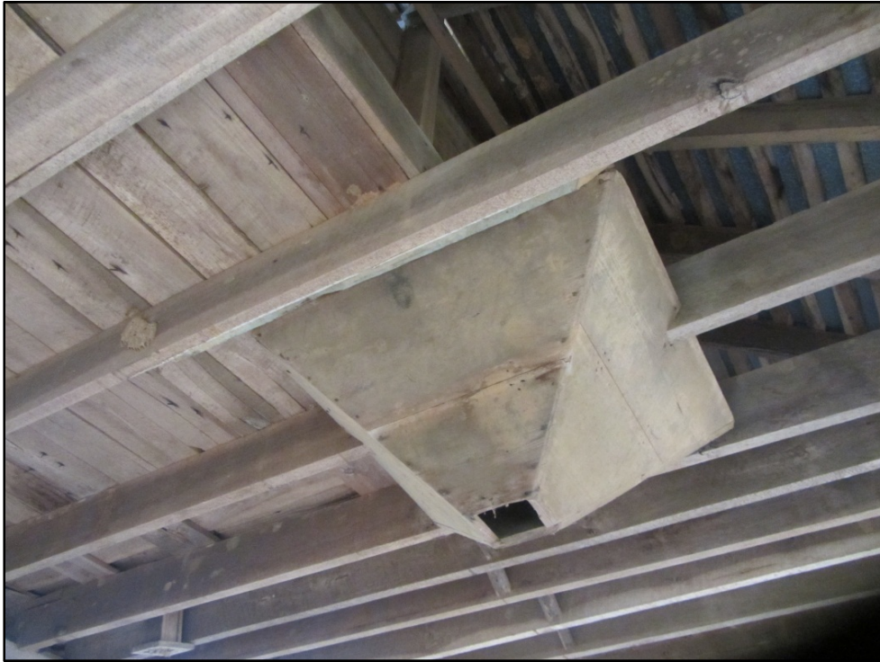
Figure 23. Ward Mill (AM 457), detail of original grain hopper hanging from ceiling on second floor.
