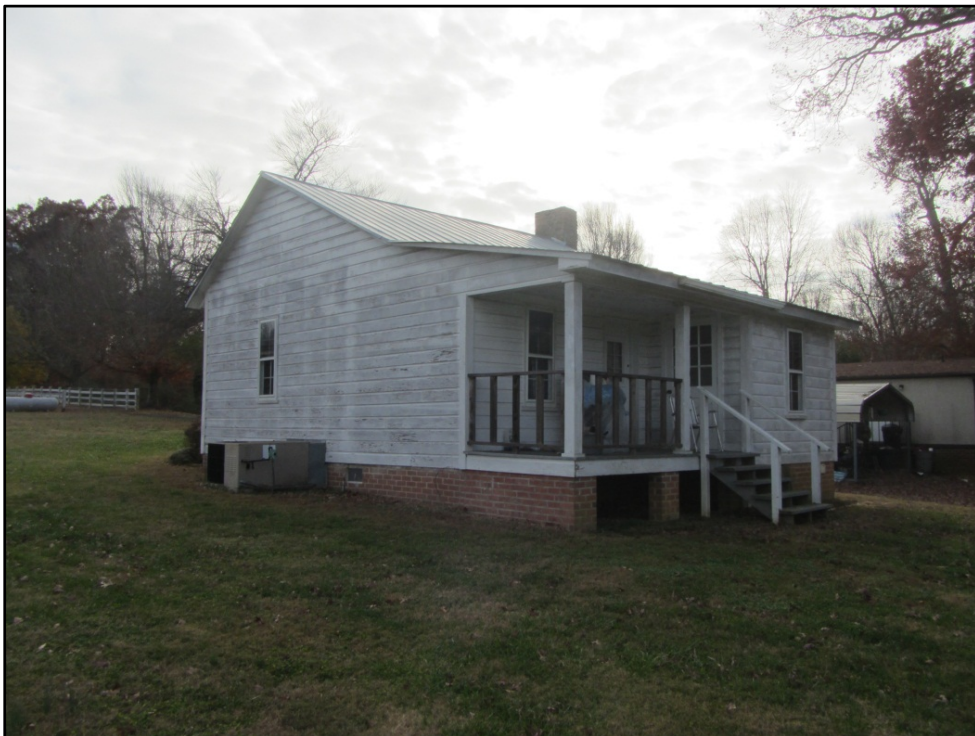
Figure 28. Ward Mill House (AM 458), northeast corner of house, looking southwest.
