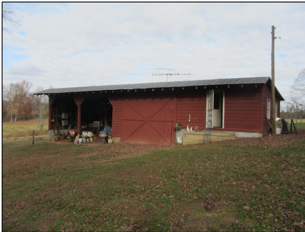
Figure 32. Vehicle Shed #1, looking northeast from mobile home.
