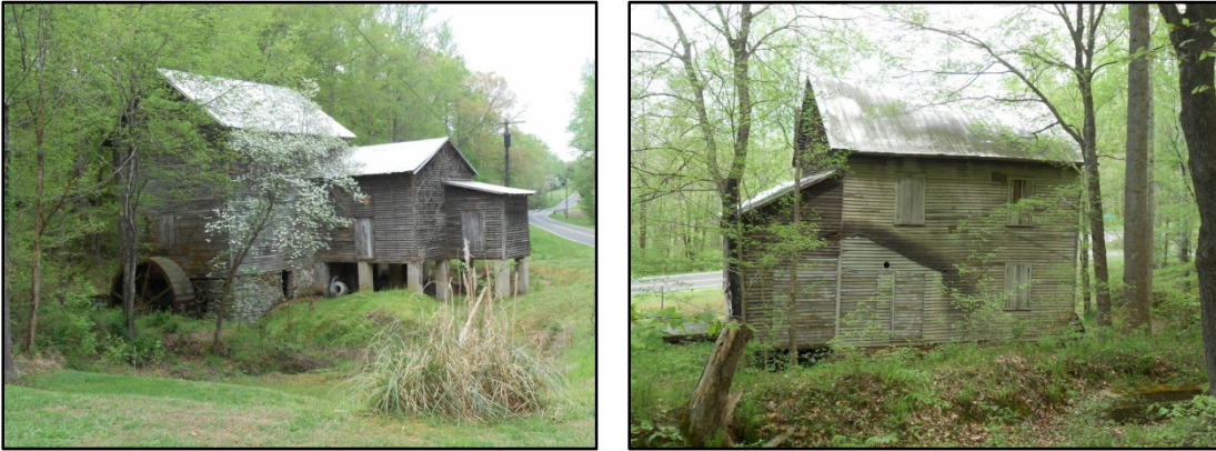
Figure 39. Two views of Cook's Mill.
