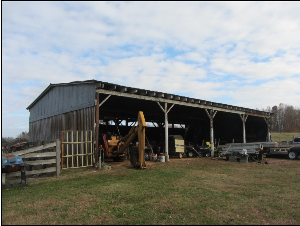
Figure 33. Vehicle Shed #2, west façade, looking southeast from driveway.
